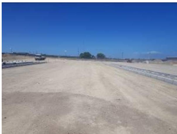
Image 32: Compacted area, awaiting paving.
