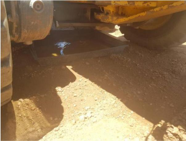
Image 16: Drip tray placed under stationary construction vehicle.
