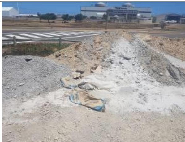
Image 30: Cement bags not disposed of correctly.
