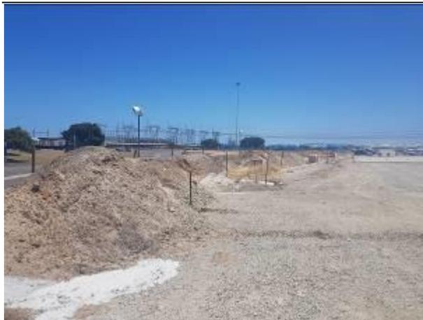
Image 29: Topsoil stockpile for rehabilitation.
